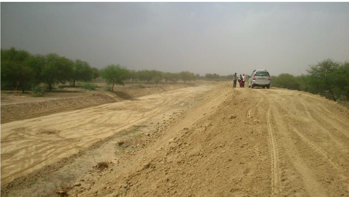
Near to Completion
