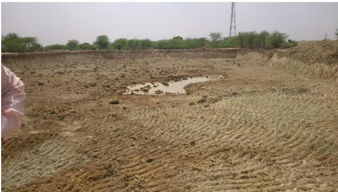
Near to Completion
