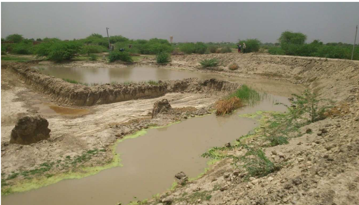
Near to Completion
